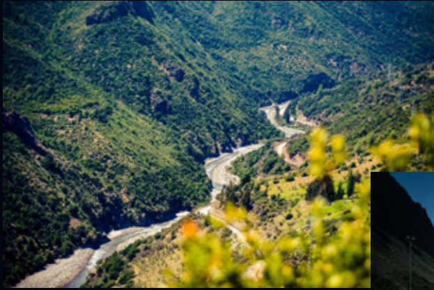
Hydroelectric project in Chile.
